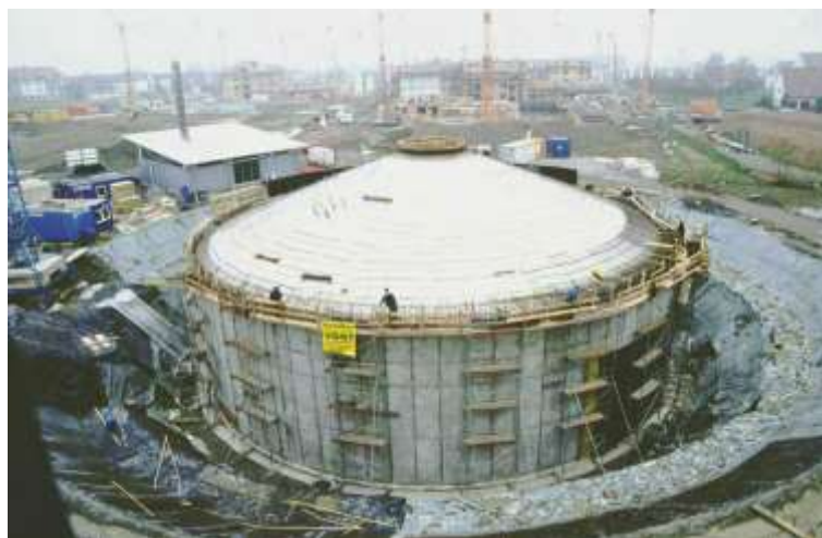
Figure: Construction of a big TTES (12,000 m 3 ). Friedrichshafen (Germany, 1996)
