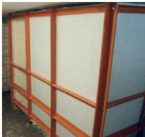
Figure: Hot water storage tanks. (Source: Universitat Stuttgart)
