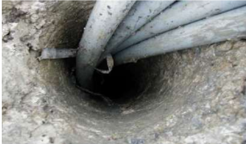
Figure: Geothermal borehole (source: Solites)
