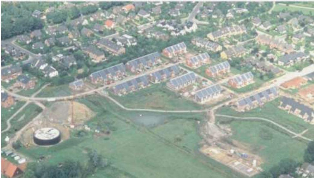
Figure: Central solar heating plant with seasonal storage (CSHPSS) in Hamburg (1996) (Source: Solites)
