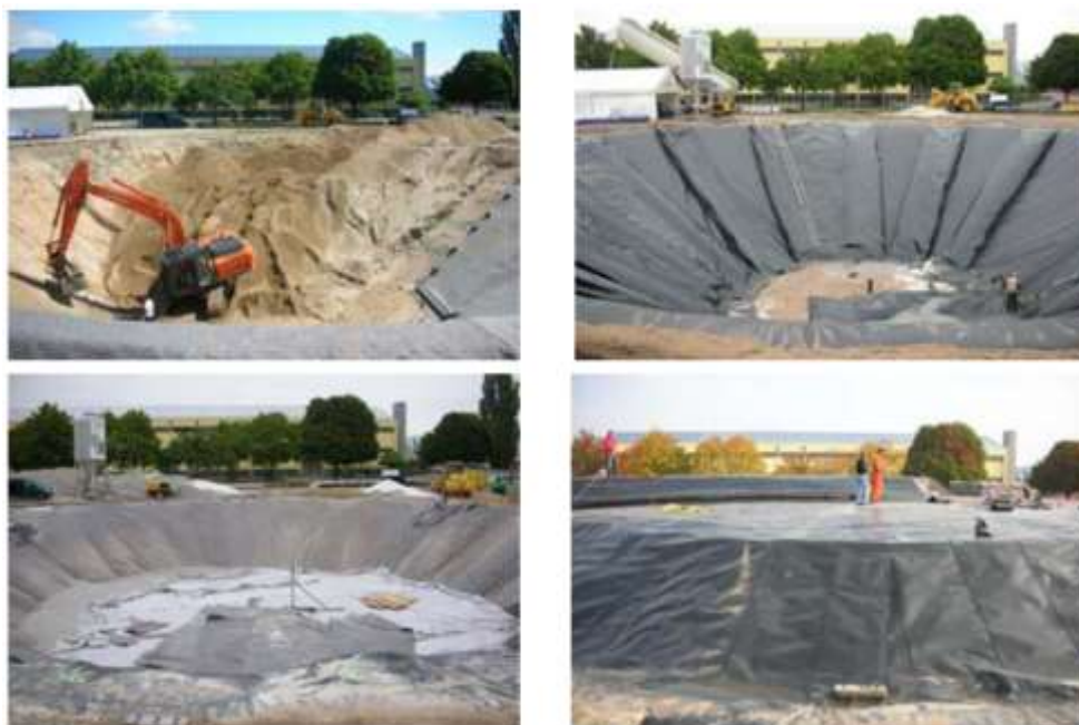
Figure: Pit storage construction in Eggenstein, 2008 (4,500 m 3 ).
