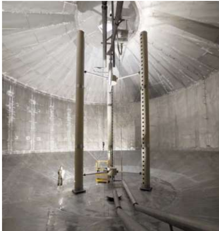
Figure: Internal aspect of a big TTES (6,000 m 3 ). Ackermannbogen (Munchen)
