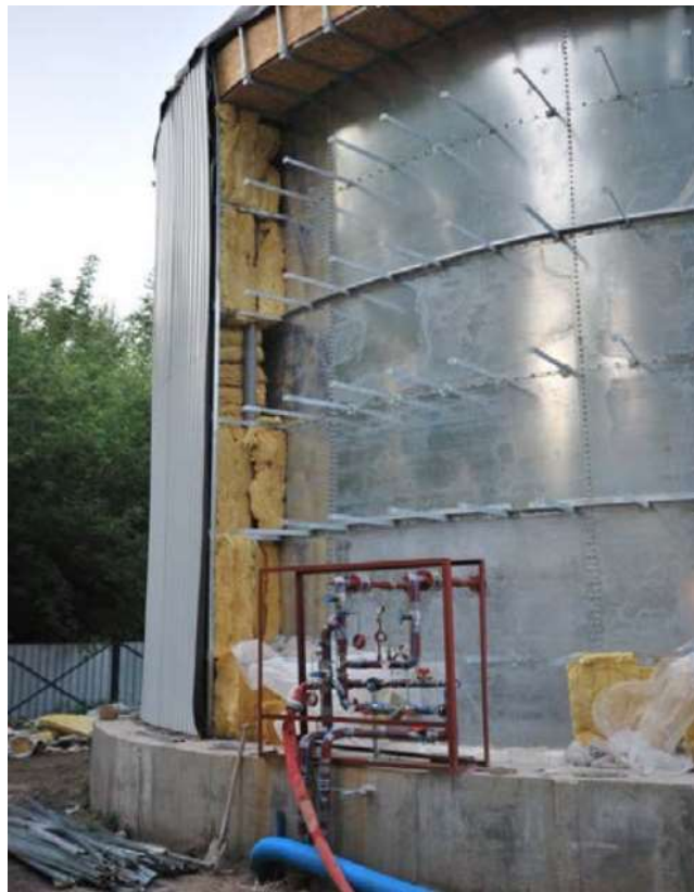
Figure: Seasonal thermal storage (800 m 3 ) in Zabki (Poland). It is visible the great thickness isolation of the wall (70 cm). (Source: Einstein Project)
