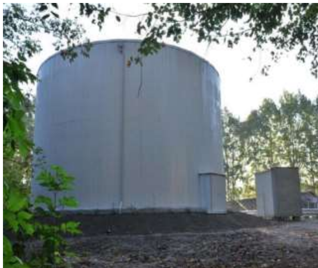
Figure: Seasonal thermal storage during operation. October 2014 (Source: Einstein Project)
