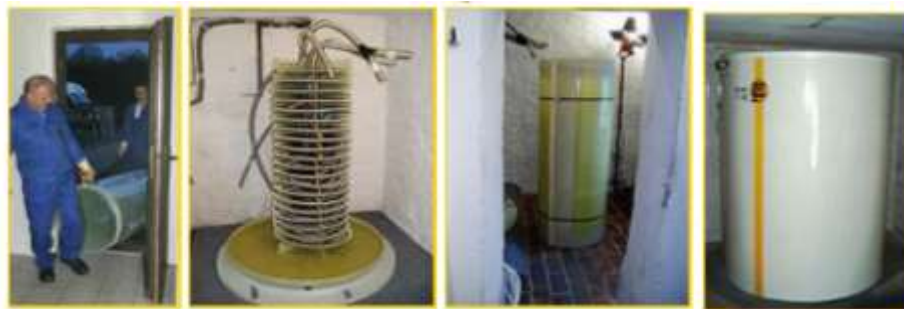
Figure : T400's construction technique (Source: Haase, Haase-Wärmespeicher)
