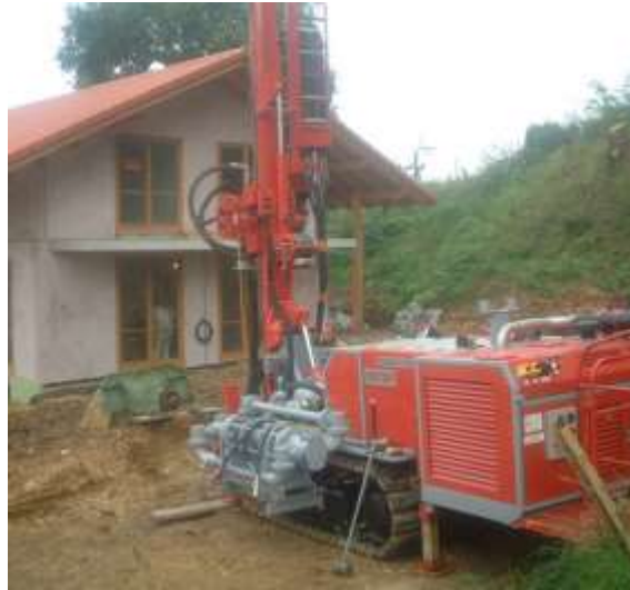
Figure: Rotary Drilling (Source:hdengineering)
