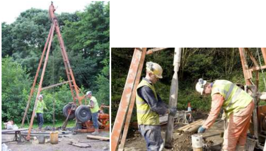
Figure: Cable percussion drilling (Source: RSA Geotechnics)
