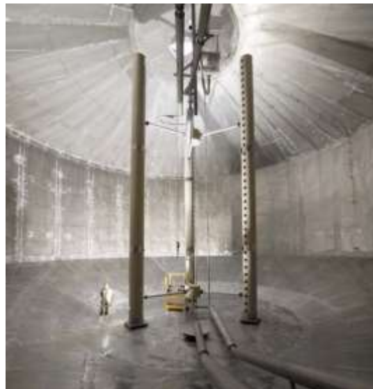
Figure: Internal aspect of a big TTES (6,000 m 3 ). Ackermannbogen (München)
