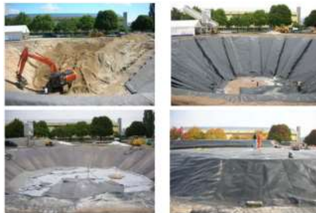
Figure: Pit storage construction in Eggenstein, 2008 (4,500 m 3 )(Source: D2.1).
