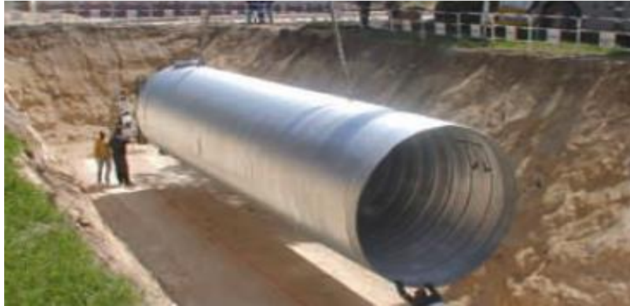
Figure: Corrugated Steel Pipes (Source: BCT, SPIRosol)
