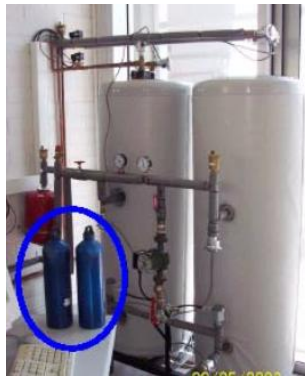
Figure: PCM modules included in domestic hot water tanks (Source: D2.1)
