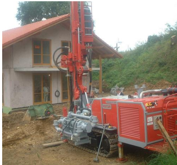
Figure: Rotary Drilling (Source:hdengineering)
