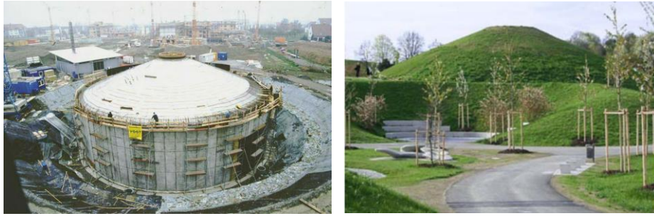
Figure: Construction of a TTES in Germany and integration of a TTES into the landscape (Source D2.1)
