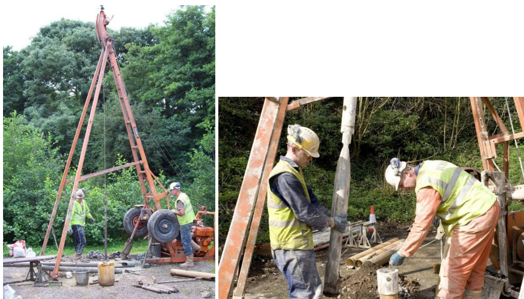
Figure: Cable percussion drilling (Source: RSA Geotechnics)
