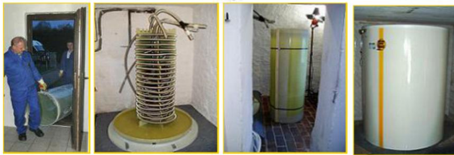
Figure : T400's construction technique (Source: Haase, Haase-Wärmespeicher)
