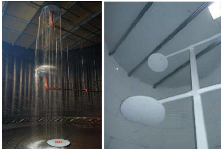
Figure: Stratification devices for the Einstein Project
