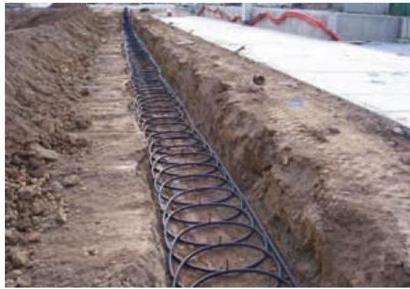
Figure: Slinky Horizontal (Source:IDAE)
