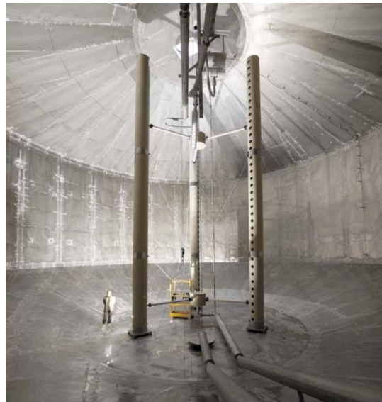
Figure: Internal aspect of a big TTES (6,000 m 3 ). Ackermannbogen (Munich)
